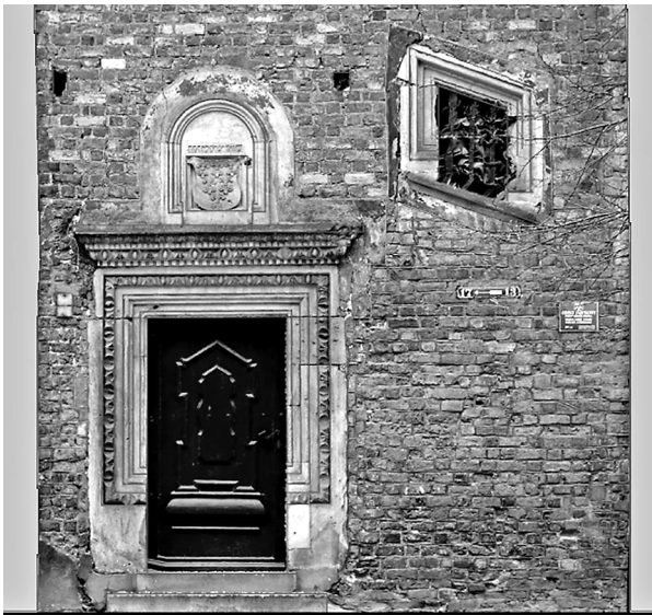
Fig. 9. Example of orthophoto delivered from 3D mesh model with some overlaying 2D vector lines. Medieval chapter-house in Wrocław (Poland)
