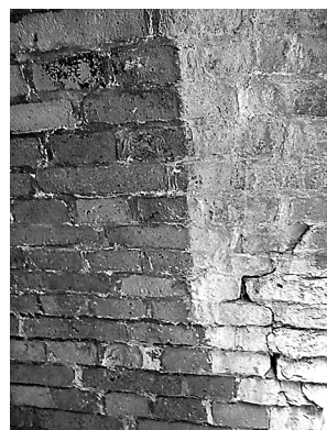
Fig. 15. Surface of bridge before cleaning
