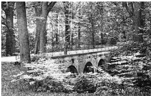
Fig. 9. Arcade Bridge (beginning of 20th c.)
