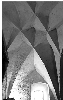
Fig. 2. “Cell Vault” in Trebsen (Germany), where the curves, surfaces and also the masonry textures could be surveyed and analyzed (D. Wendland)
