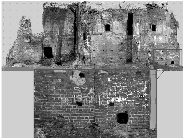
Fig. 6. Example of colour (RGB) orthophoto acquired directly from 3D point cloud. Southern façade of mediaeval bishop palace in Milicz (Poland)
