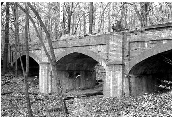
Fig. 2. Royal bridge (before 1999)
