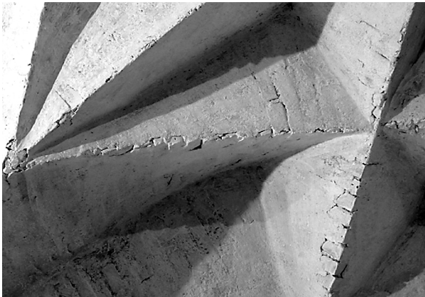
Fig. 9. Due to the continuity of the masonry texture, the courses are not arranged perpendicular to all groins, as usually assumed. Such observations lead us to understand the construction principles and rules applied by late Gothic masons (D. Wendland)
