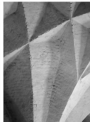
Fig. 3. Detail of the analyzed vault, showing the geometric complexity of the curve described by the inward fold, and the continuity of the masonry texture; both in contrast to the current description model (D. Wendland)
