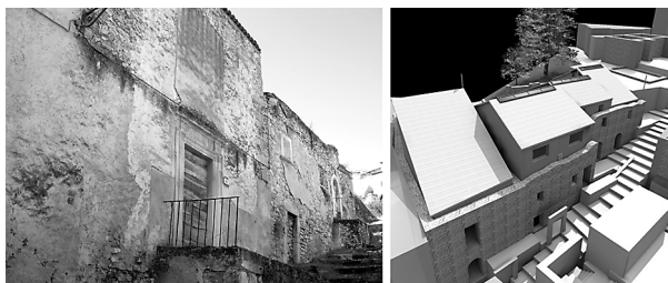
Fig. 4 The masonry buildings before and after the rehabilitation works
