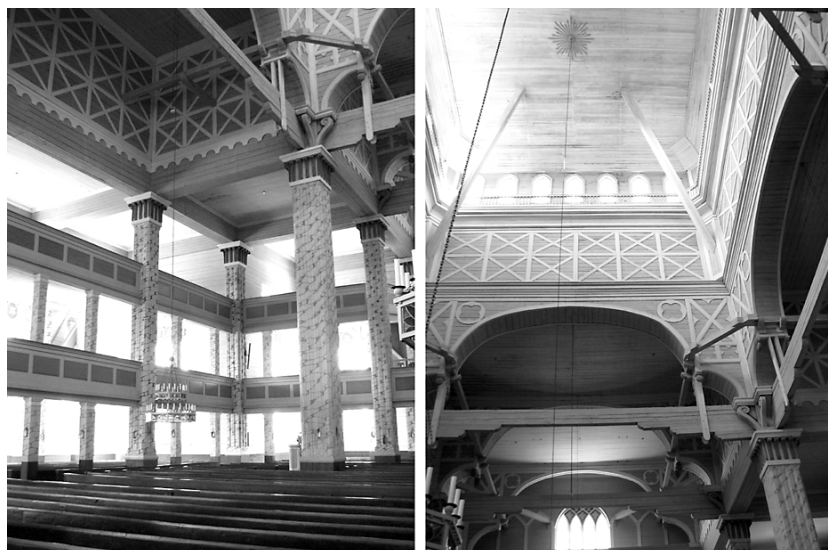
Fig. 10-11. The pillars are reinforced by richly profiled tie-beams connected to the walls (Photo Anu Soikkeli, 2011)
