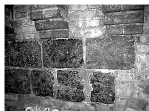
Fig. 17. Arcade Bridge – built-in original structural elements made of glass slag
