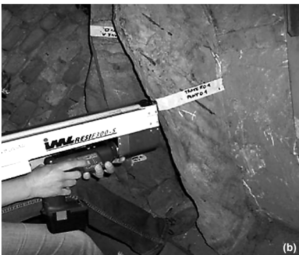
Fig. 8. Sampling of the wooden structure for identification: from the joist (a); from the rib (b); and from the reed mat (c)
