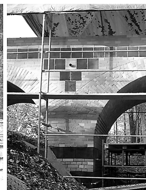
Fig. 16. Surface of bridge after cleaning
