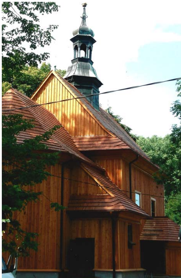
Ryc. 16. Widok na kościół od strony prezbiterium i zakrystii (pn-wsch..) po zakończeniu prac, lipiec 2012 r. Fig. 16. View of the church from the side of the presbytery and sacristy (north-east) after completing the work, July 2012
