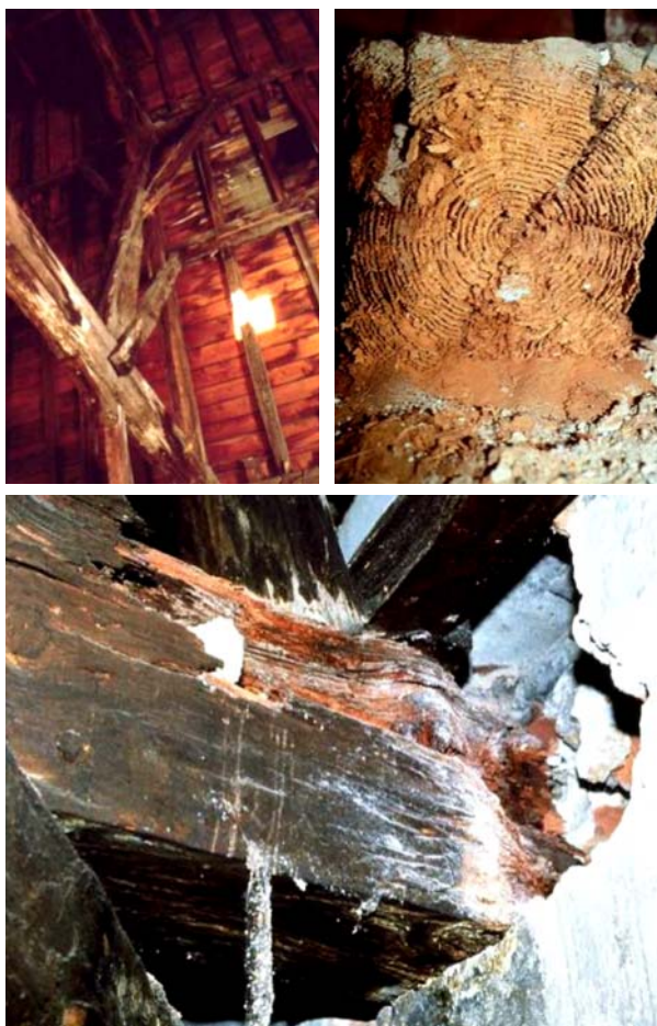
Figs. 8–10. Biotic decay due to due fungi and insects (photo C.B. 1986)
