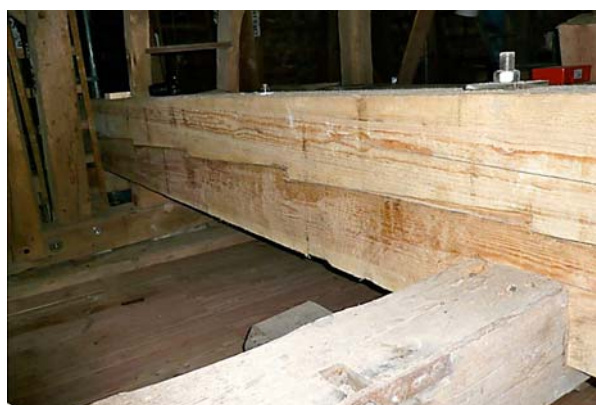
Fig. 3. Left: 270 years old teathed beams as upstand beams; right: true to original reproduced teathed beam (wood species: pine)
