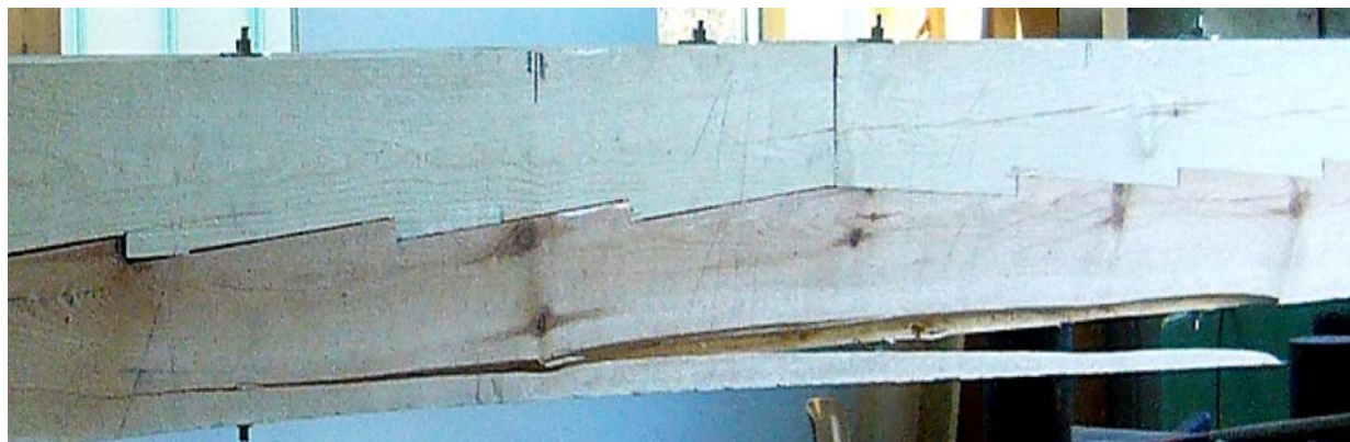
Fig. 11. Specimen 01 – tensile fracture on the bottom surface
