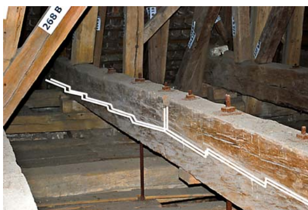
Fig. 3. Left: 270 years old teathed beams as upstand beams; right: true to original reproduced teathed beam (wood species: pine)
