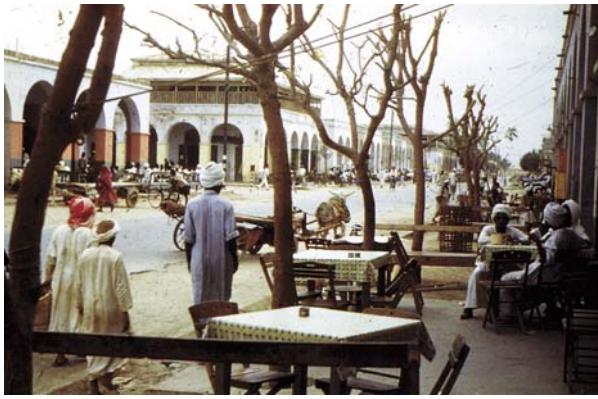
Fig. 1. Old Khartoum Street. Photo: [in:] Authors' Archive
