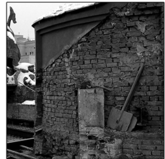
Coursed brick masonry of the early 20th century (The House with Chimaeras)
