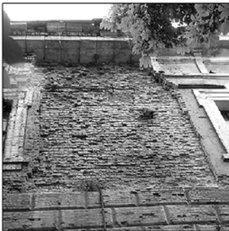
Coursed masonry of red brick of the 19th century (Mystetskyi Arsenal)
