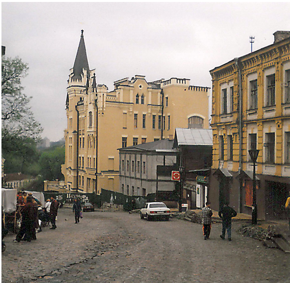
Fig. 4. Residential house at 15 Andriivsky Uzviz Str. Photo by Julia Ivashko, 2017
