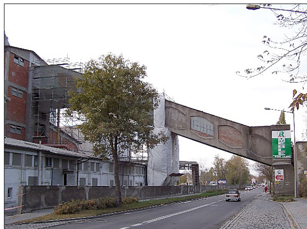
Fig. 2. View of the reinforced concrete flyover, 2007; photo by D. Bajno
